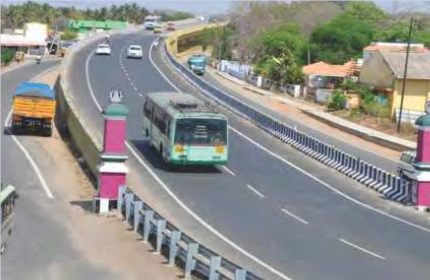
Railway Over Bridge at Ottanchatram, Dindigul District, inaugurated by the Hon'ble Chief Minister of Tamil Nadu on 24.02.2014
