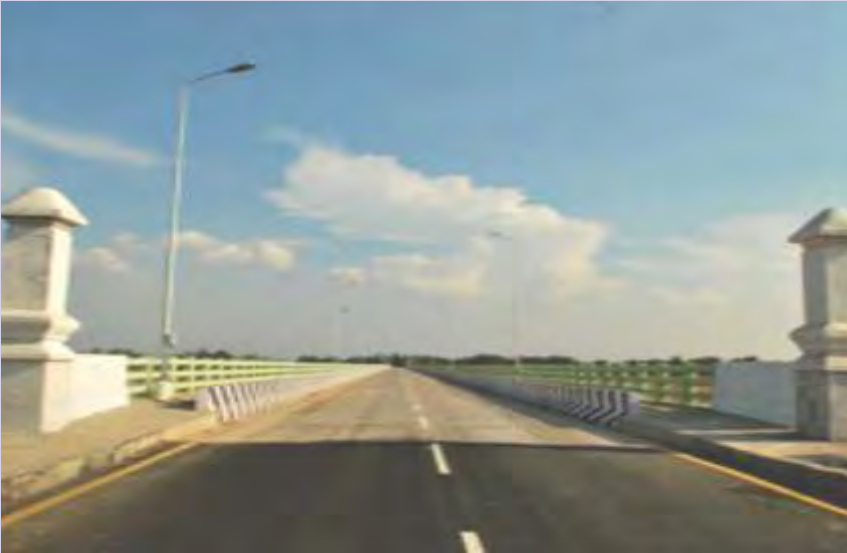
High Level Bridge at Pazhamarneri, Thanjavur District inaugurated by the Hon'ble Chief Minister of Tamil Nadu on 12-06-2014
