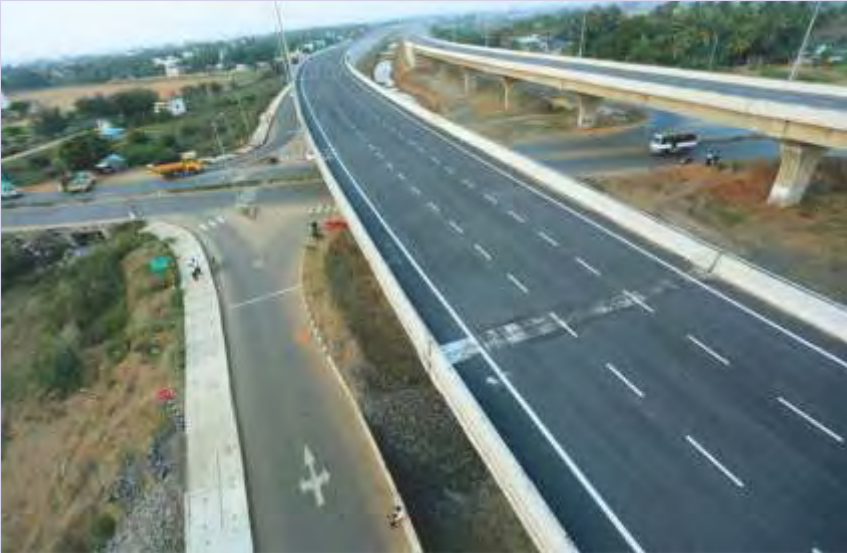
Mannivakkam Flyover constructed across SH-48 in Chennai Outer Ring Road
