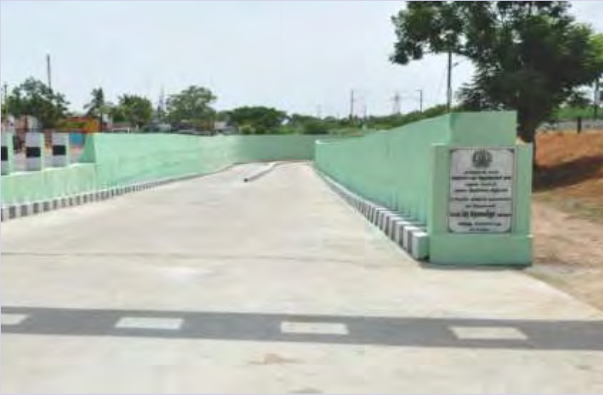
Limited Use Subway at Paravai, Madurai District inaugurated by the Hon'ble Chief Minister of Tamil Nadu on 12-06-2014.
