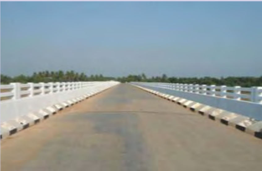
High Level Bridge at Murugankudi, Kilimangalam in Cuddalore District inaugurated by the Hon'ble Chief Minister of Tamil Nadu on 12-06-2014.
