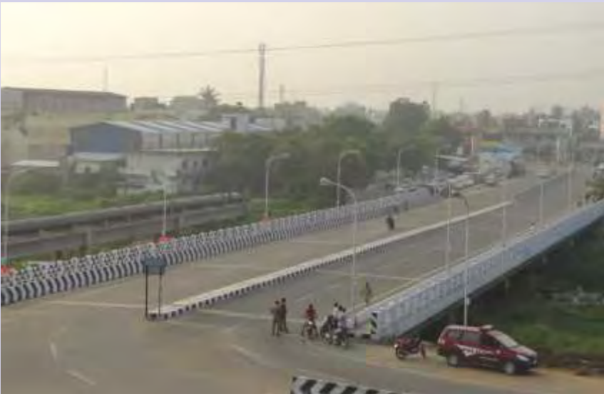
High Level Bridge at Nerkundram, Chennai inaugurated by the Hon'ble Chief Minister of Tamil Nadu on 11-11-2013.
