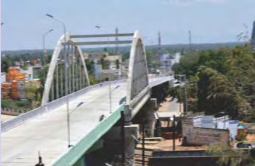
Railway Over Bridge at Tenkasi, Tirunelveli District, inaugurated by the Hon'ble Chief Minister of Tamil Nadu on 11.11.2013.
