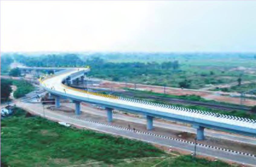
Railway Over Bridge at Ulundurpet, Villupuram District, inaugurated by the Hon'ble Chief Minister of Tamil Nadu on 11.11.2013
