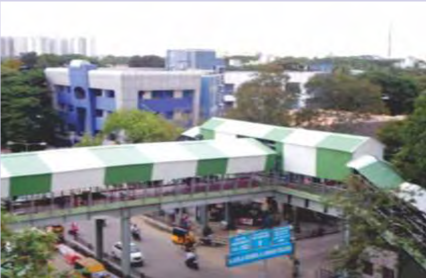
Foot Over Bridge on Chennai Inner Ring Road near SBOA School Junction inaugurated by the Hon'ble Chief Minister of Tamil Nadu on 12-06-2014.
