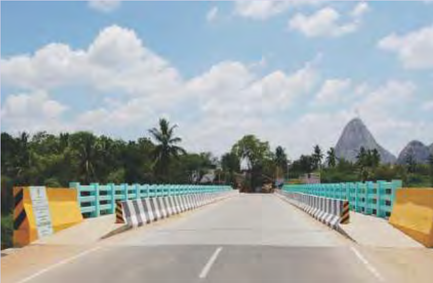
High Level Bridge at Ervadi in Tirunelveli District inaugurated by the Hon'ble Chief Minister of Tamil Nadu on 24-02-2014.
