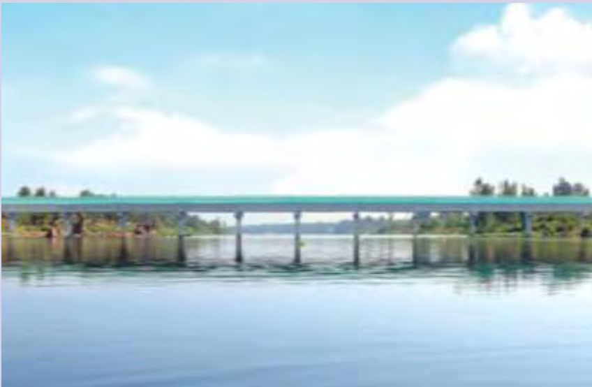
High Level Bridge between Kokkarayanpettai in Namakkal and Lakkapuram in Erode District inaugurated by the Hon'ble Chief Minister of Tamil Nadu on 24-02-2014
