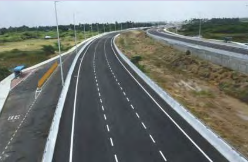
View of Amudhurmedu Busbay in Chennai Outer Ring Road
