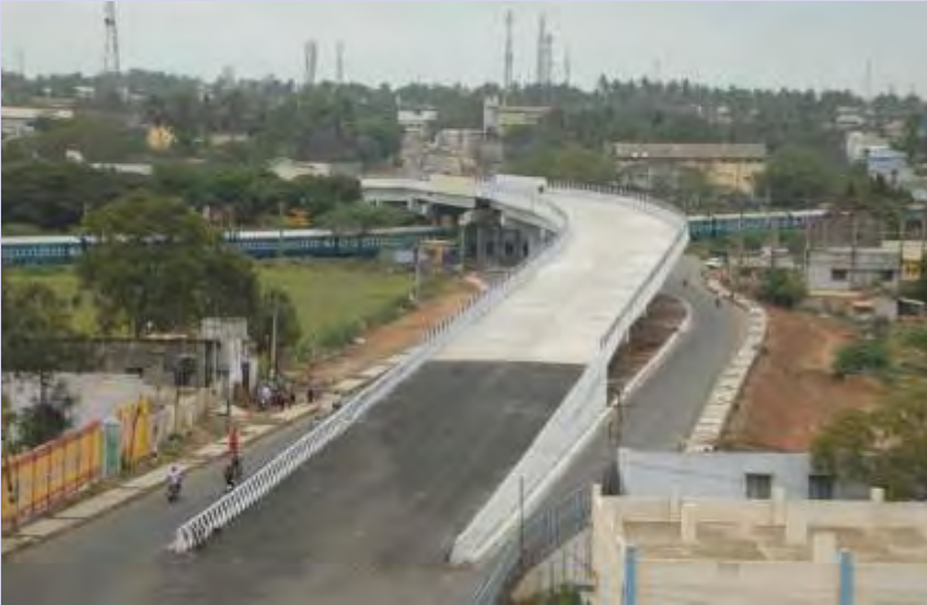
Railway Over Bridge at Echanari, Coimbatore District inaugurated by the Hon'ble Chief Minister of Tamil Nadu on 11-11-2013
