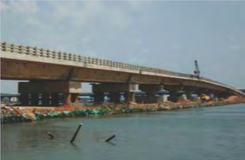
High Level Bridge at Ennore creek, Tiruvallur District inaugurated by the Hon'ble Chief Minister of Tamil Nadu on 24-02-2014
